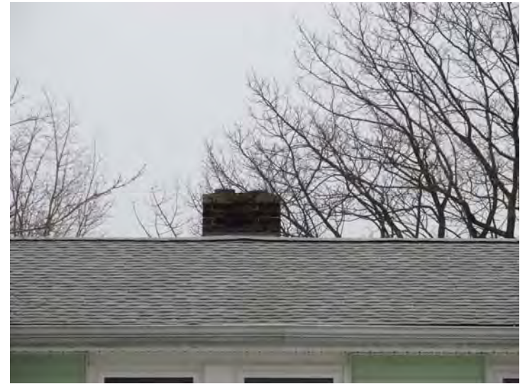
Newer architectural shingles on some buildings are in good condition
