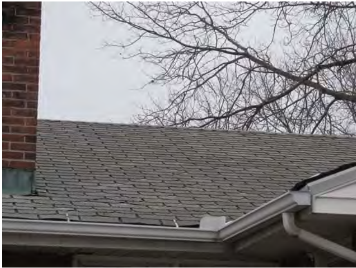
Older three-tab shingles on some roof surfaces exhibit significant wear and deterioration
