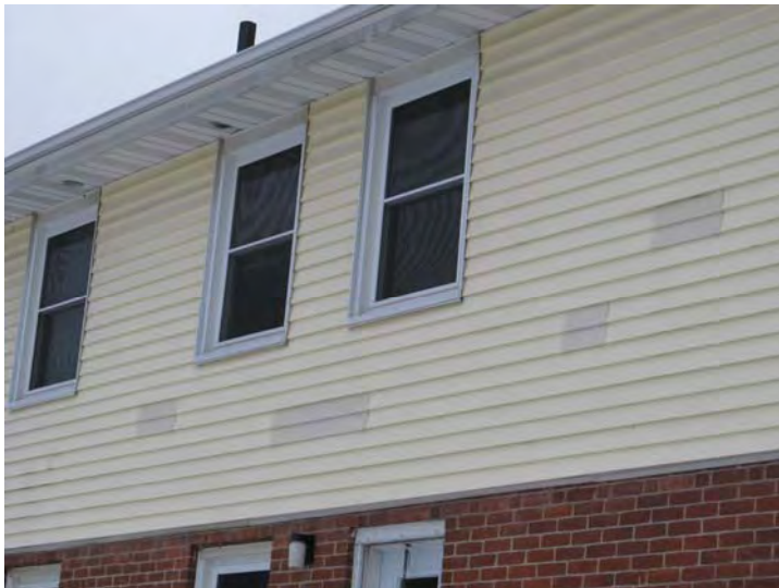
Vinyl siding exhibits areas of past patch repairs at various locations
