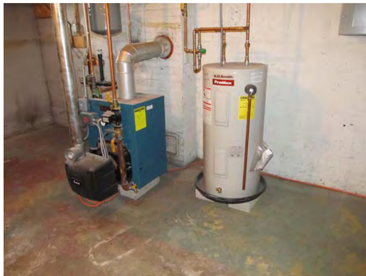
Newer unit-level boiler for generation of hydronic heat and adjacent indirect-fired domestic hot water tank – Future domestic hot water tanks will be freestanding electric models
